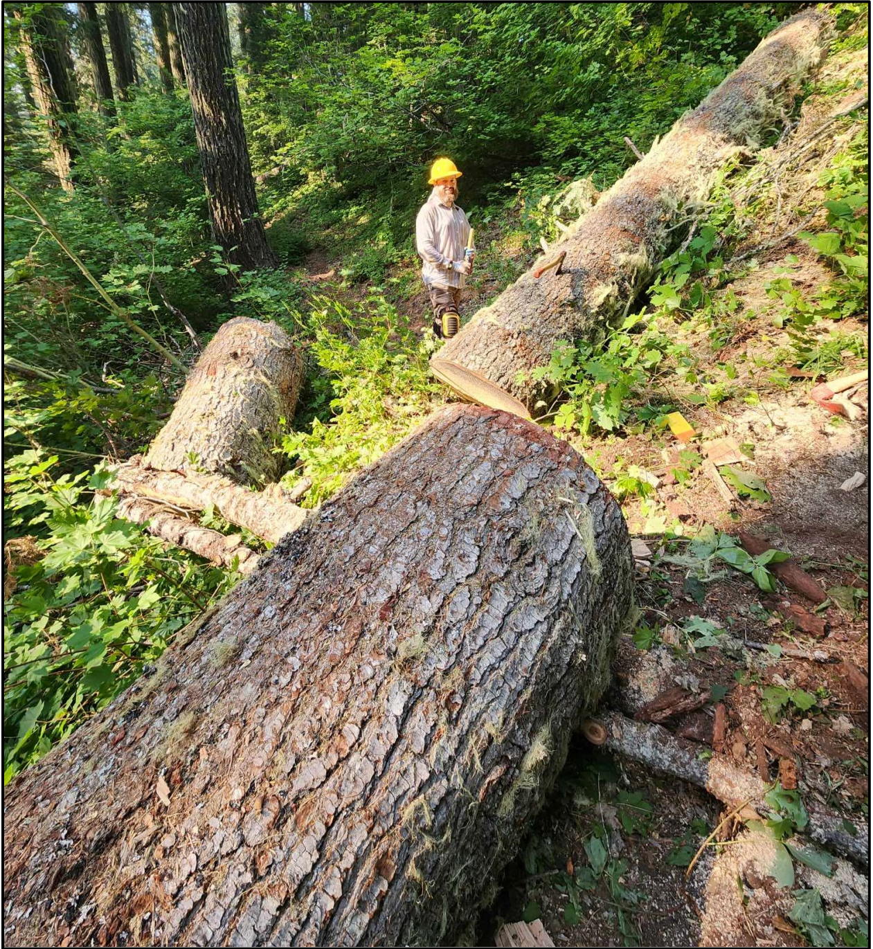
Figure 8: Once the grand fir at mile marker 1.4 was bucked, it began to slide over a blowdown into the trail. It required a second cut to allow pedestrian and equestrian passage.
