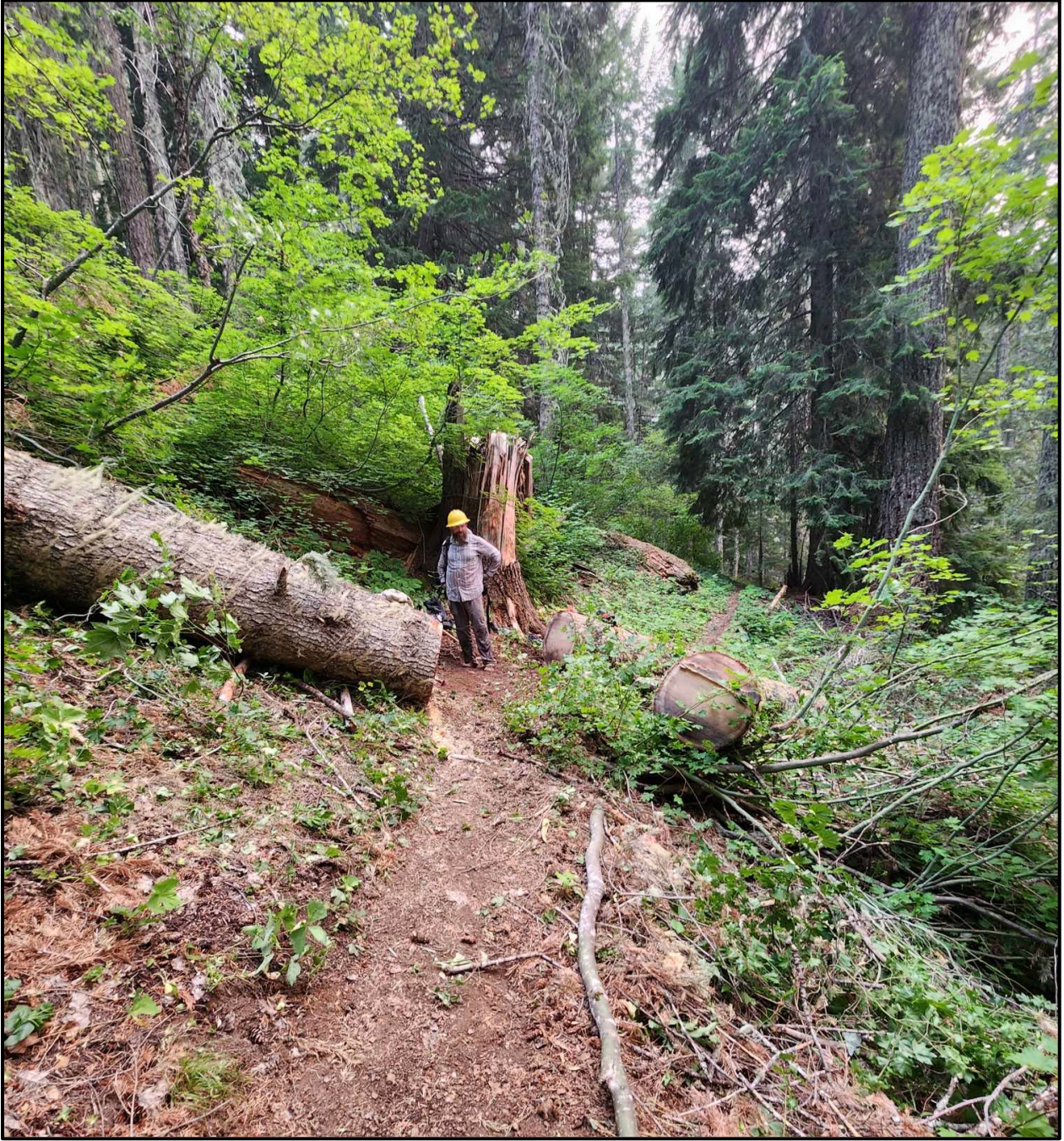
Figure 9: Project completion at mile marker 1.4.
